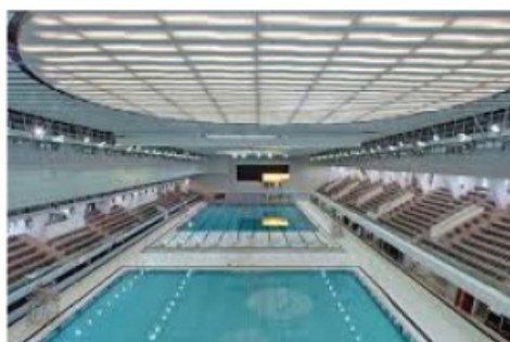
New main and multi-purpose pools inside the complex
