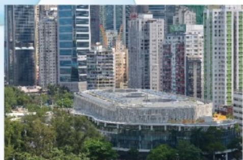
Exterior of the new Victoria Park Swimming Pool Complex
